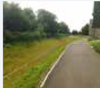
Footpath/Cycleway and Swale
