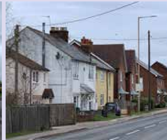
Medium density housing on Station Road
